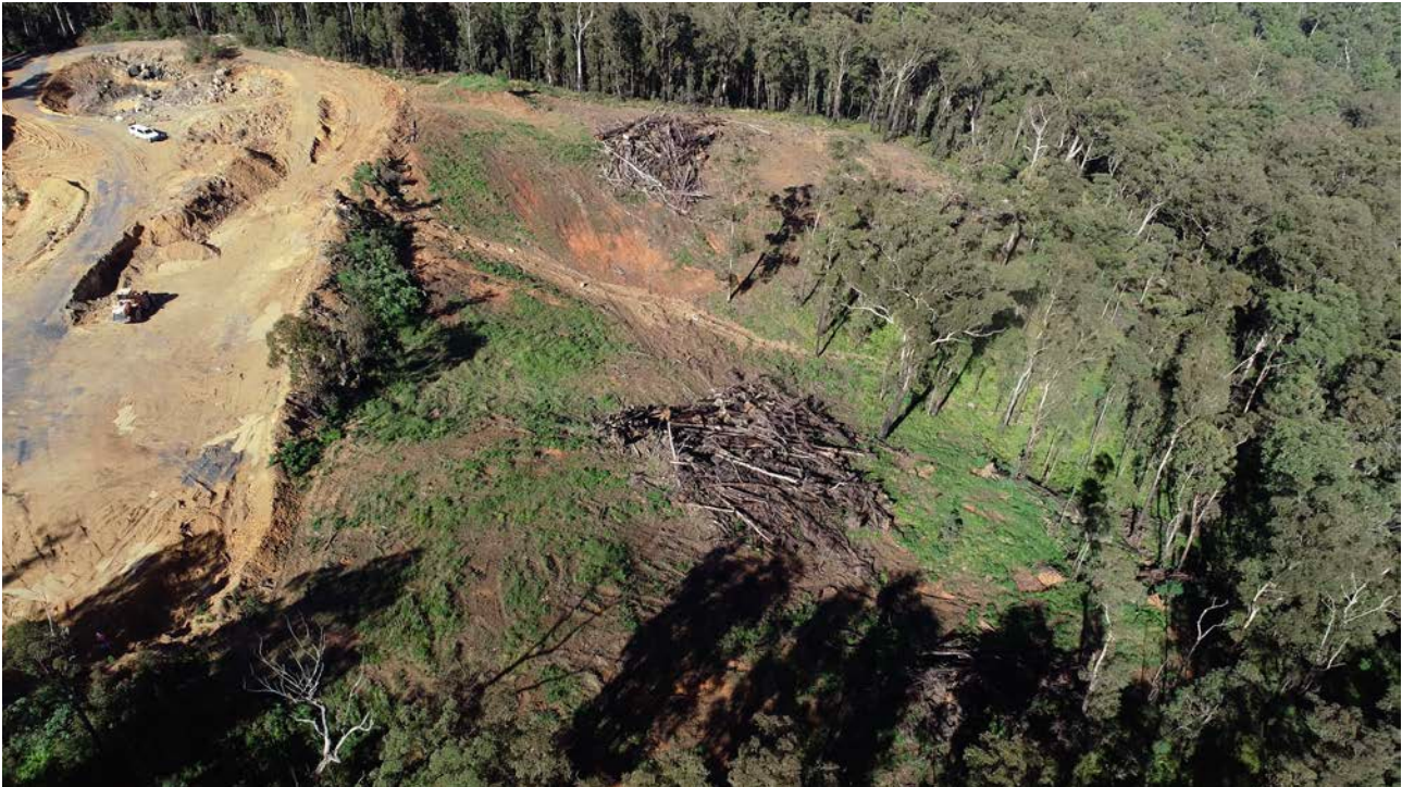
PHOTOGRAPH 3.2: Oblique drone photograph of cleared area below the existing quarry proposed for lateral expansion (centre and right hand side). View looking west
