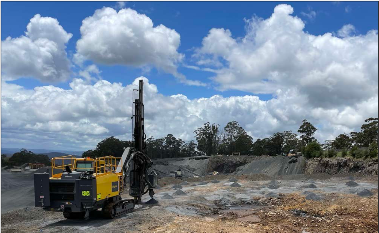
PHOTOGRAPH 3.3: Drill rig in the process of drilling holes for blasting at Sheridans Hard Quarry operation at Hernani
