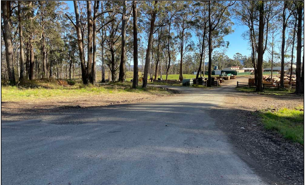
PHOTOGRAPH 7.4: Sealed section of quarry access route from Armidale Road
